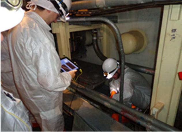
Fig. 1. Engineers Performing IM Testing of Cables Installed in Reactor Containment
